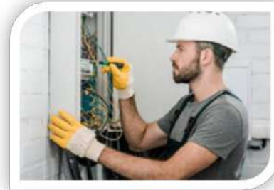
5+ Distribution box inspection
