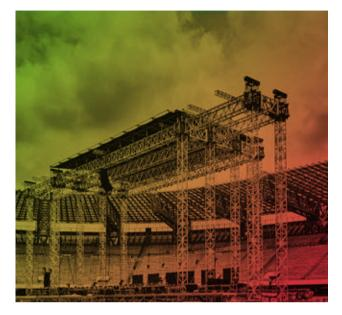
The Roof size can easily be adapted by combining the width (33, 30 and 27 meters) and the depth (20, 17 and 14 meters). In any formation, the towers in conjunction with the ballast base system guarantee high stability and solidity of the structure.
