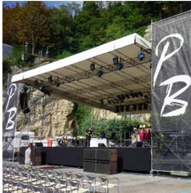
Square section heavy duty aluminium truss twist-resistant version with 40 cm long sides.
