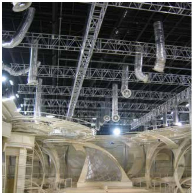
Rectangular section High Load aluminium truss with 76 x 52 cm long sides. It is diagonalized on all faces and is provided with steel fork connections. It ensures high load capacity on medium-long spans thanks to the design of its main components.
