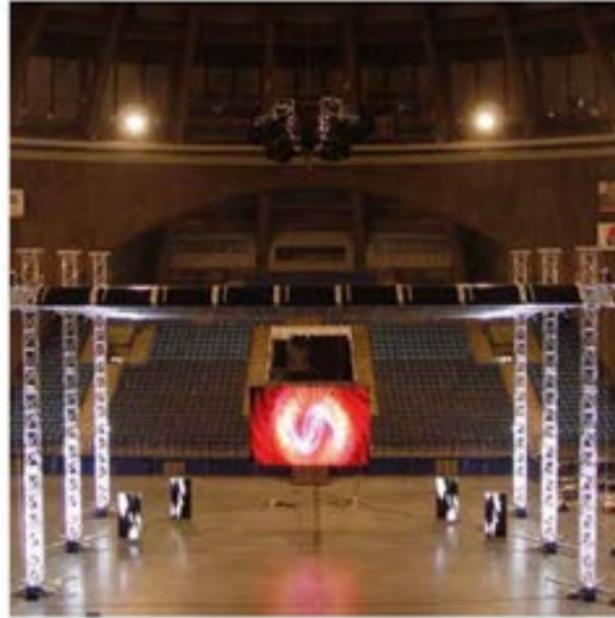
LIBERA is an open structural system. Roof systems in LIBERA 76 consist of Maxitowers and a LIBERA FL76 grid structure. For the double-pitch version normal LIBERA FL76 trusses are used with the addition of support systems and sliding guides for the roofing sheet, which are fixed to the grid. This arrangement has the advantage of having a horizontal hanging plane.
