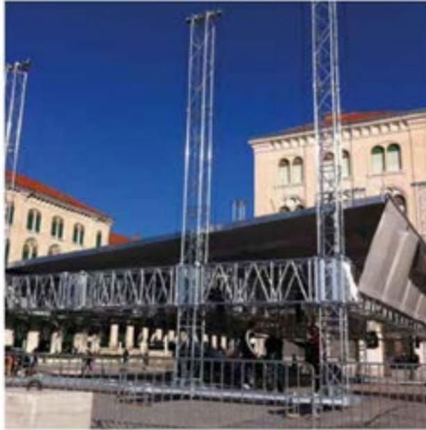
High Load roof systems are particularly suitable for medium-sized covered structures. They consist in load bearing trusses with universal fork connections for high-end solutions.
