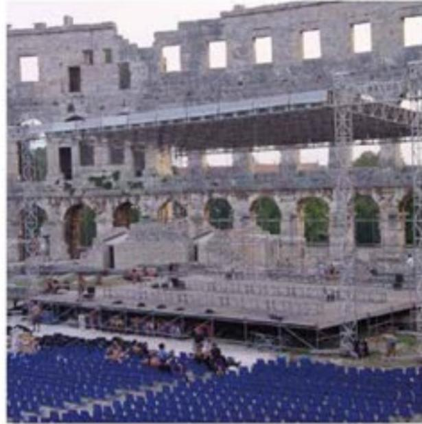
Designed for small to medium events, the single pitch 10x8 m roof covers your needs perfectly. The use of QX30SA truss for the towers and Qx40SA truss for the roof provide a safe and sturdy structure that handles your more demanding loads.
