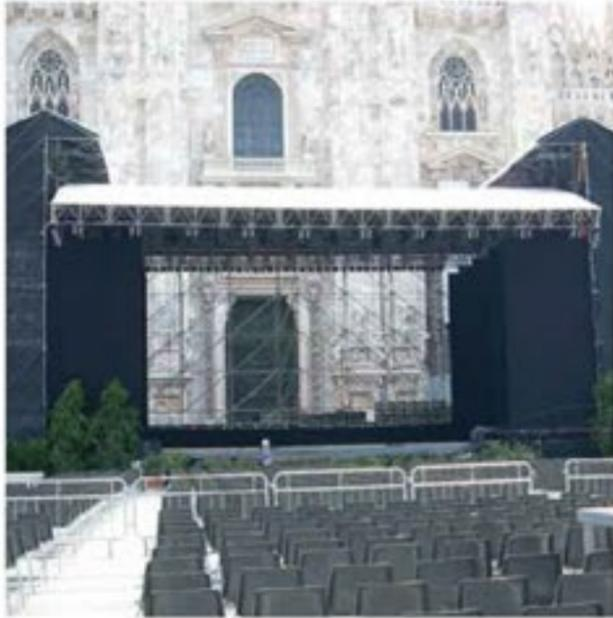
LIBERA is an open structural system. Roof systems in LIBERA 76 consist of Maxitowers and a LIBERA FL76 grid structure. With the single-pitch roof, the upper grid structure consists of trusses with built-in LIBERA FL76R roofing sheet guides.
