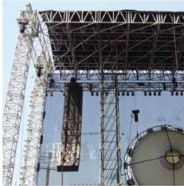
This is the largest roof system in the LIBERA range, and one of the biggest and best performing on the market. It is based on the LIBERA concept and consists of Maxitower 76 and LIBERA FL105 trusses. It is imposing and sturdy, and is – in itself – the most spectacular element of the show. The structure has excellent technical specifications and is highly modular.
