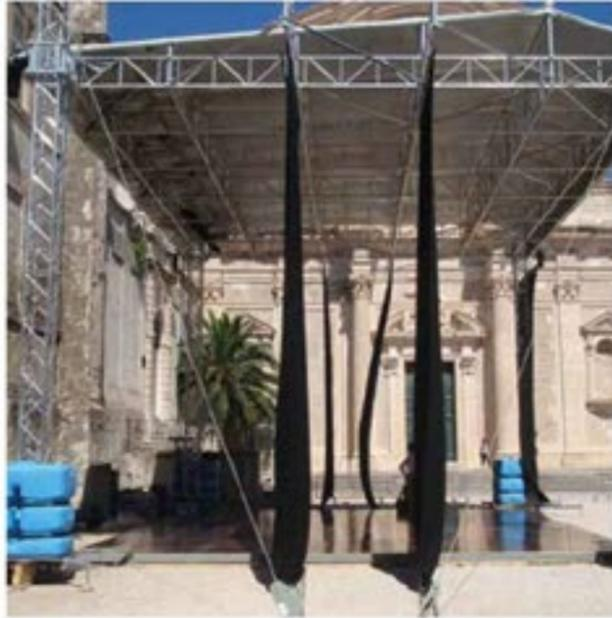
LIBERA is an open structural system. Roof systems in LIBERA 52 consist of Maxitowers and a LIBERA FL52 grid structure. The actual span can reach 16 metres, to which side wings may be added.
