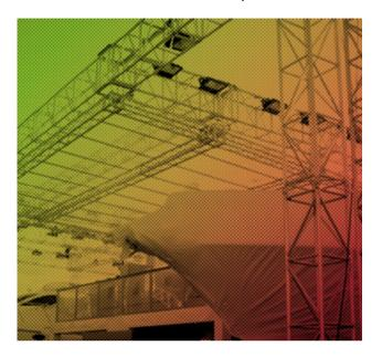
These roof systems are high-performance structures that feature a connection made through steel forks. This line was designed when a high loading capacity is required together with wide spans.
