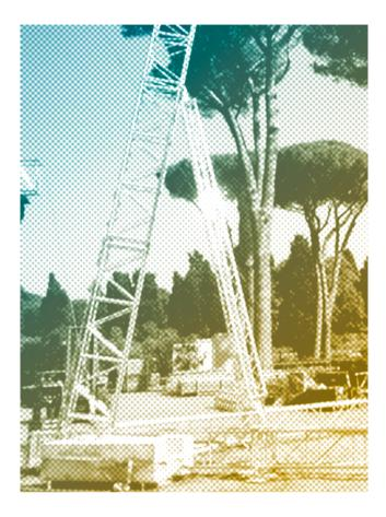
Support tower for for audio systems. Designed in QL40A, this new Flyintower is suitable for 1,600 kg loads and can reach the height of 10 meters, thus ensuring sturdiness and rigidity on relevant heights. It also utilized QH30SA trusses as stabilizing elements and is equipped with fork connections.
